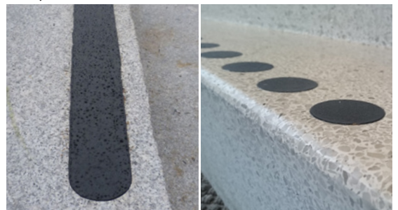
Raised circle markings on stairs.
