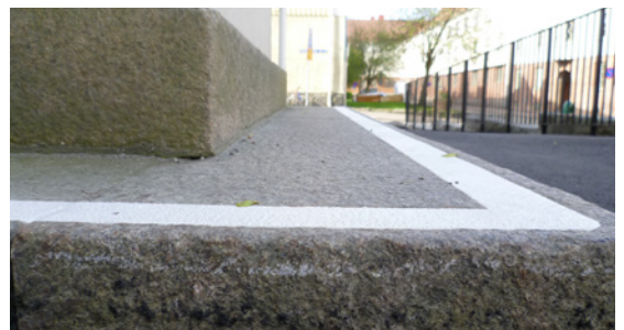
Sunken contrast marking line, available in both white and black (see below).
