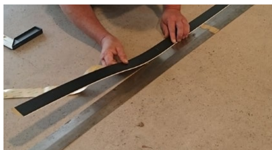
After exact measurement, carefully remove the covering paper from the reverse side of the strip.
